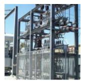
A Metal-Enclosed Bank comes fully assembled, tested, and ready for interconnection. No field assembly is required. Therefore, installation costs and problems associated with mistakes during installation are very low.
