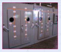
**Switching Devices:** In switched applications stages are controlled by vacuum switches, vacuum contactors, circuit breakers or other approved switching options.
